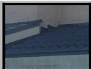
lead flashing
