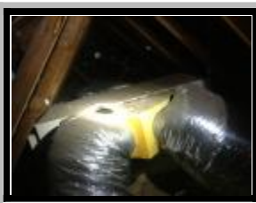
air conditioning unit
