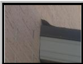
lead flashing
