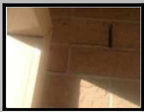
mortar joint cracked
