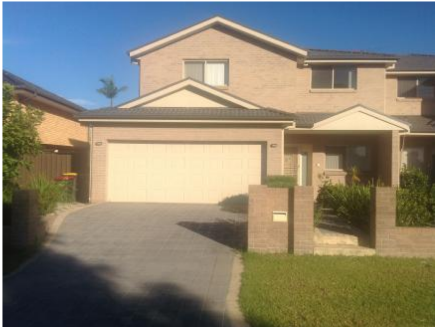
Front Elevation of the Inspected Property
