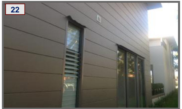
Incomplete - Flashings above windows
