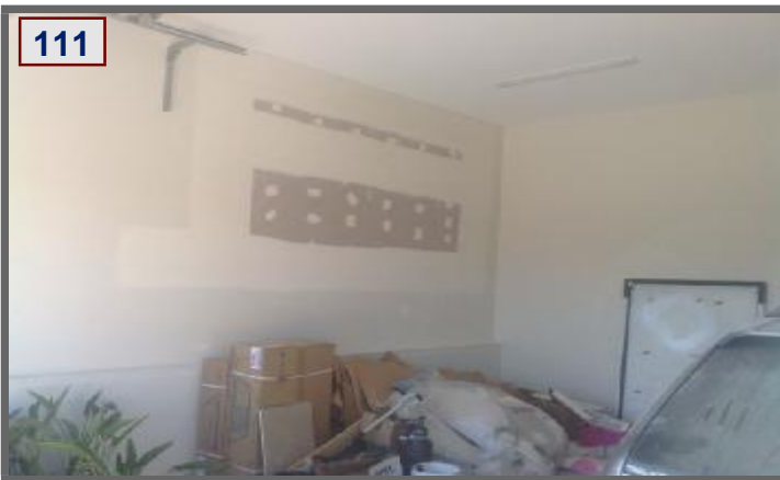
Newly plaster wall
