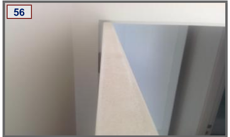
Tops & Bottoms of doors are not fully painted
