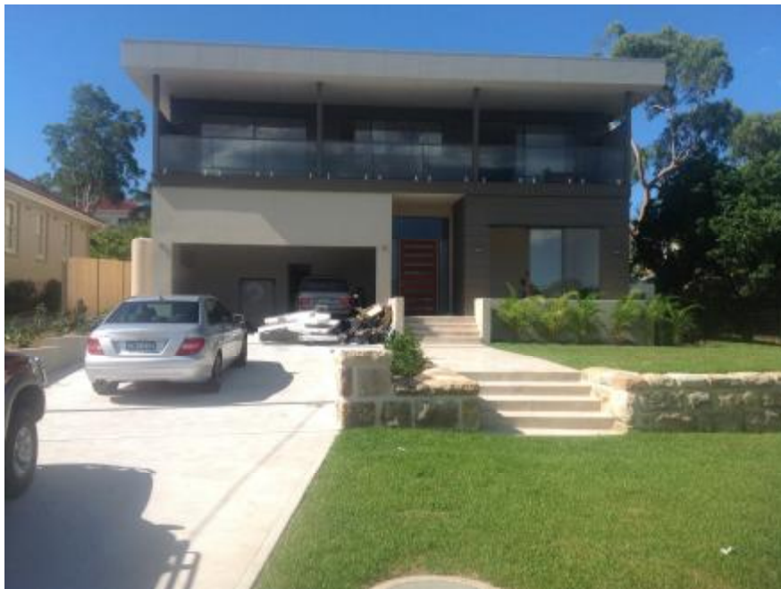
Front Elevation of the Inspected Property
