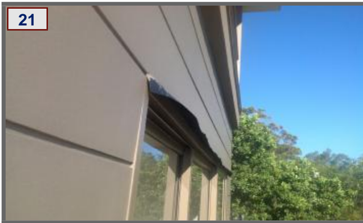
Flashings above windows - Incomplete
