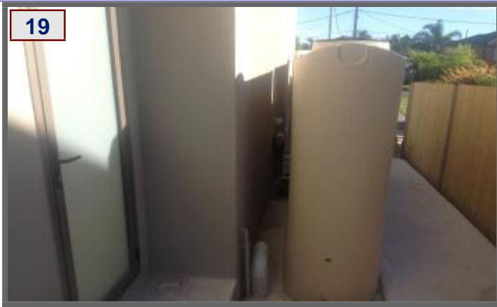
Water Storage Tank Not Installed, Incomplete render
