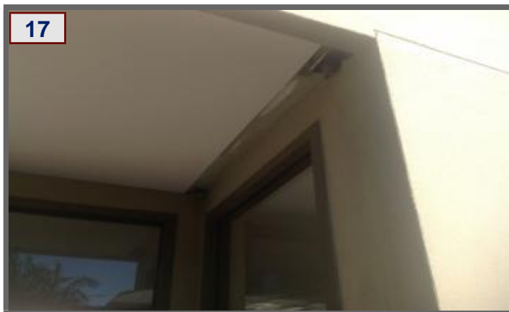
Exposed steel beam post support & nuts & bolts
