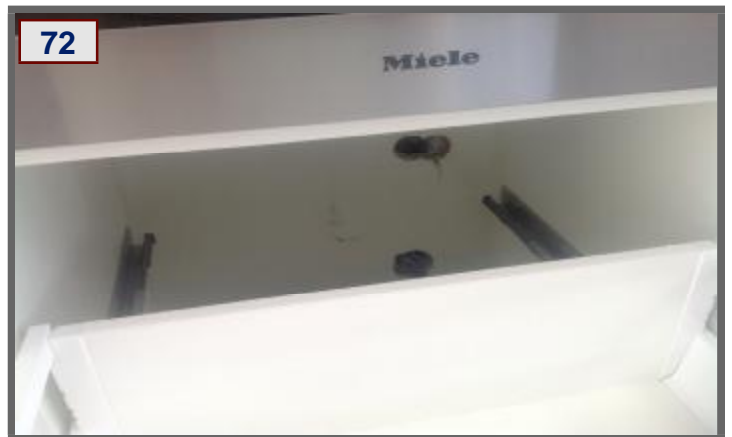
Holes in wall under oven
